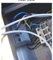
9. On WD4190 and GW4190: it is necessary to act on the mains switch TERMINALS ("Mains Switch"): maintaining, in the case of single-phase, only the phase L1 and the neutral N.
